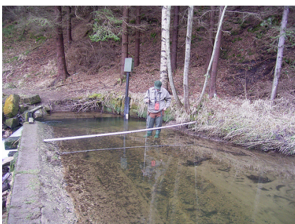
Discharge measurement station Metuje river (CZ) (above)
