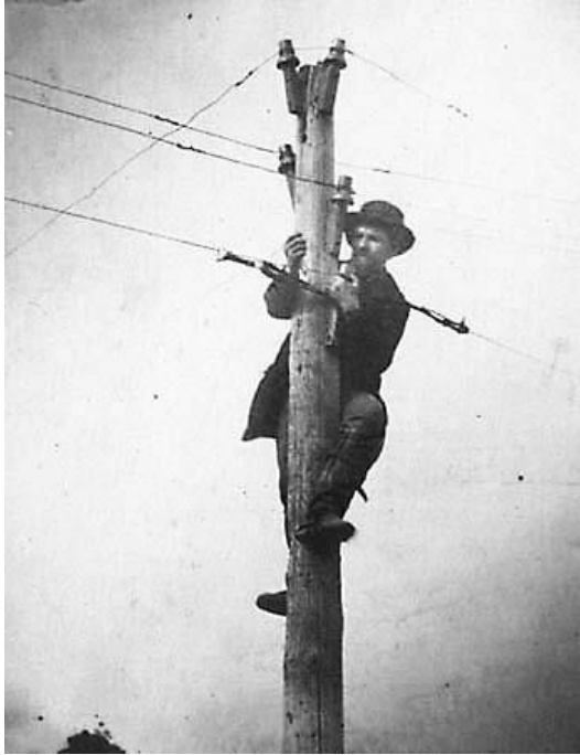
Figure 1 Telegraph sabotage: cutting telegraph wires and connecting the ends so that the point where the connection is broken cannot be detected from the ground (c. 1863).
