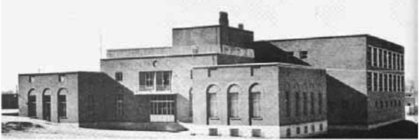
Figure 4. Original aspect of the Secondary Education building of the Instituto Escuela – JAE, from the main façade (Madrid), 1932. Carlos Arniches. (Photograph from AGA, use entitled to the author)
