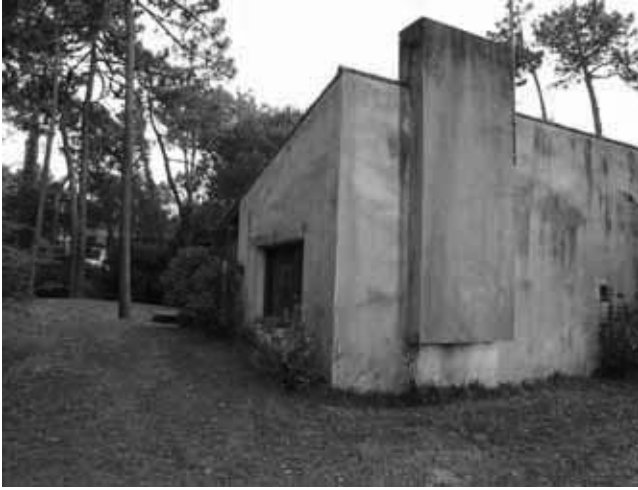
Figure 2. Partial view of the East and North facades of the Ofir House, Fao, Esposende. Fernando Távora, 1958. (Photograph by the author)
