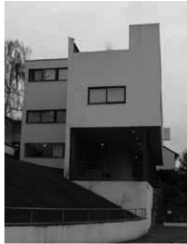
Figure 4. Le Corbusier, Double house, Weissenhofsiedlung, Stuttgart, Germany, 1927, colour photo, taken 2013
