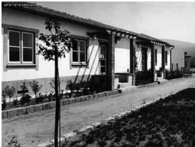
Figure 4. Arch. Joaquim Madureira, Affordable Houses Neighbourhood of Braga , 1935-39. The model developed by Raul Lino was repeated in neighbourhoods across the country until the end of 1930s. (Source: Sistema de Informação do Património Arquitectónico, http://www.monumentos.pt/ )
