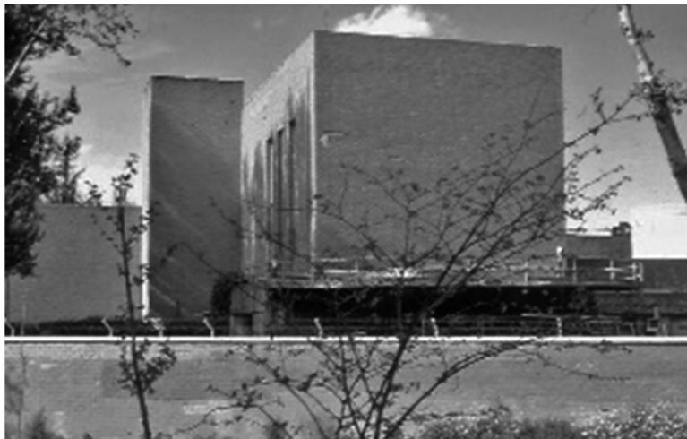
Figure 2. Central Power Station, Ciudad Universitaria (Madrid), 1932. Luis Lacasa and Manuel Sánchez Arcas. (Photograph by the author)
