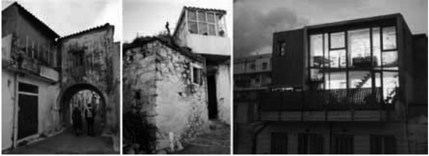
Figure 5. Small additions to houses in the villages of Pikris (Rethymnon Prefecture) and Aghios Konstantinos (Lassithi Prefecture). (The author's house in Iraklion, addition on top of an older construction, 1995-96)
