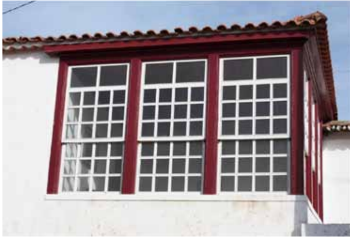
Figure 4. Transition-space. Glazed balcony in Pedrógão Pequeno © Nuno Cardoso, 2010
