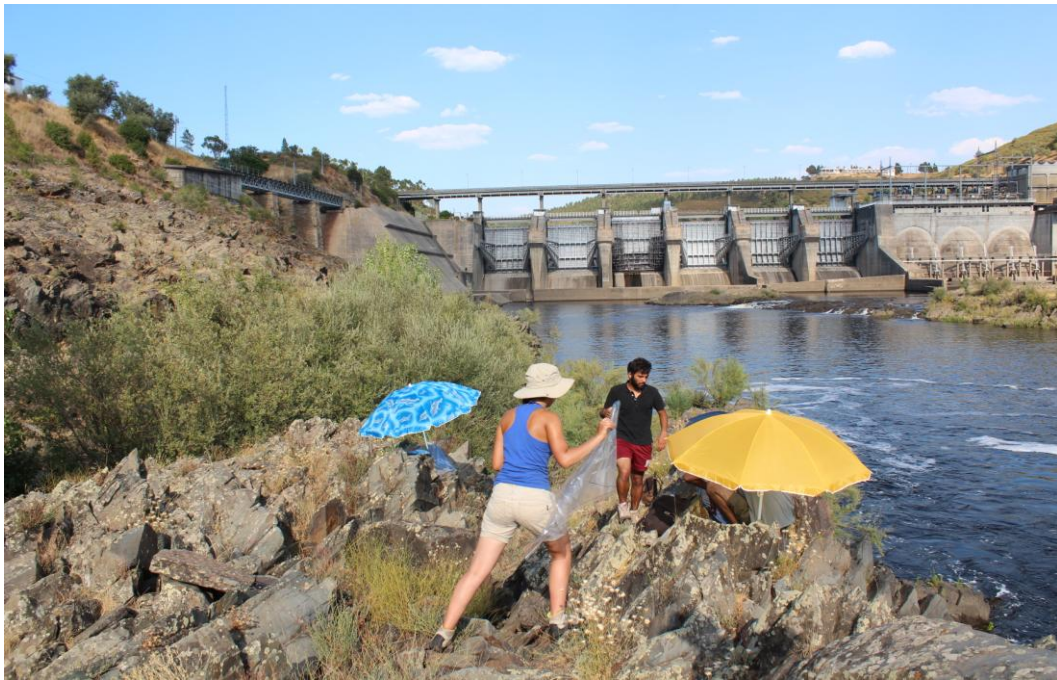
Figure 13: Image of Fratel dam facing the site of Gardete. Source: Sara Garcês 2013
