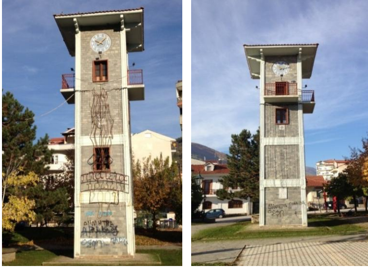
Fig. 1. Surfaces of the building
