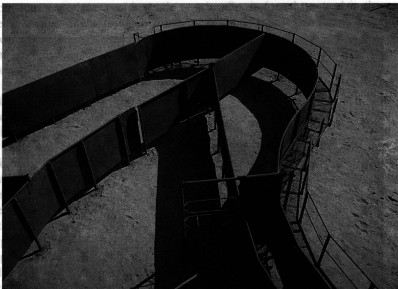
Fig. 5. Well-designed round crowd pen with solid fences and a solid crowd gate.
