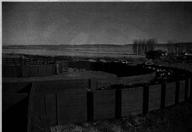
Fig. 3. Curved wood, wide curved lane with solid sides which leads to the round forcing pen.
