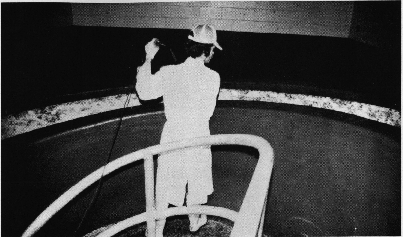
Handler works along one of the 5-ft.-radius bends in chute. Cattle move easily through curved chute with solid sides.
