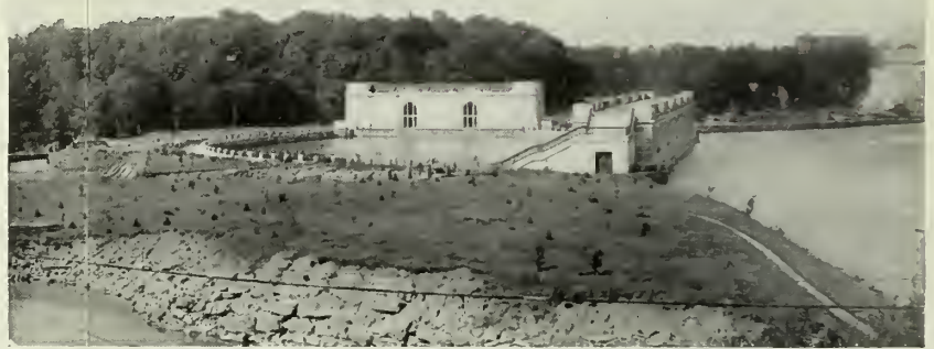
FOREBAYS, SCREEN HOUSE, AND GATE HOUSE
