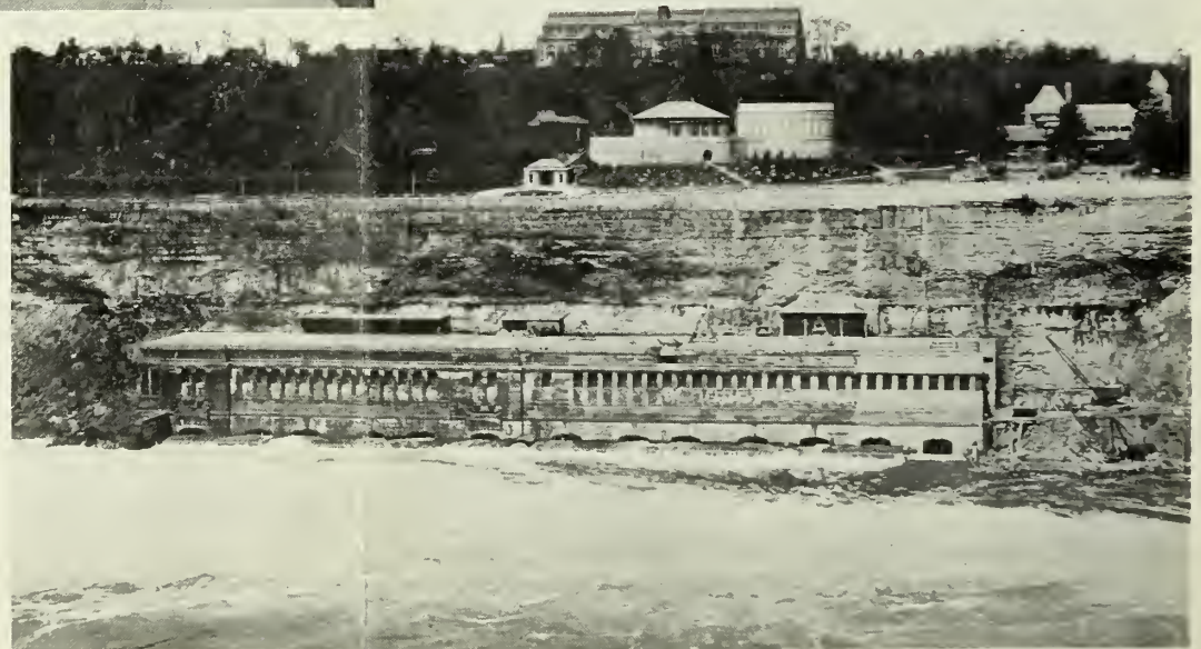
GENERATING STATION, OVERFLOW, SURGE TANK, AND DISTRIBUTING STATION AS SEEN FROM GOAT ISLAND
