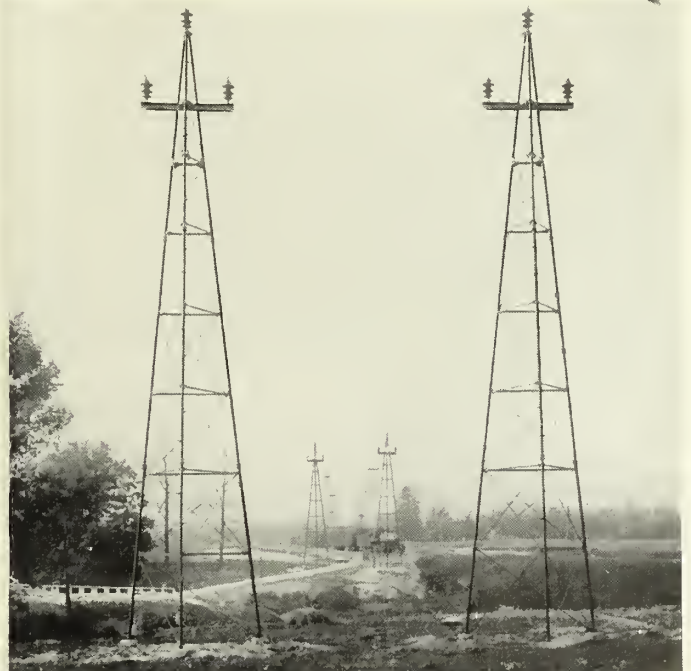
60,000-VOLT TRANSMISSION LINE — ONTARIO TRANSMISSION CO.
