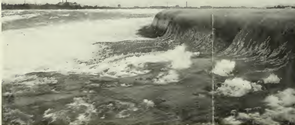
RETURN OF WATER TO RIVER OVER SUBMERGED WALL
