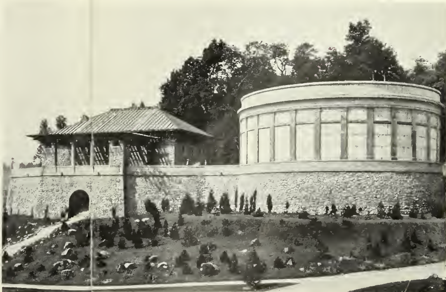
OVERFLOW AND SURGE TANK
