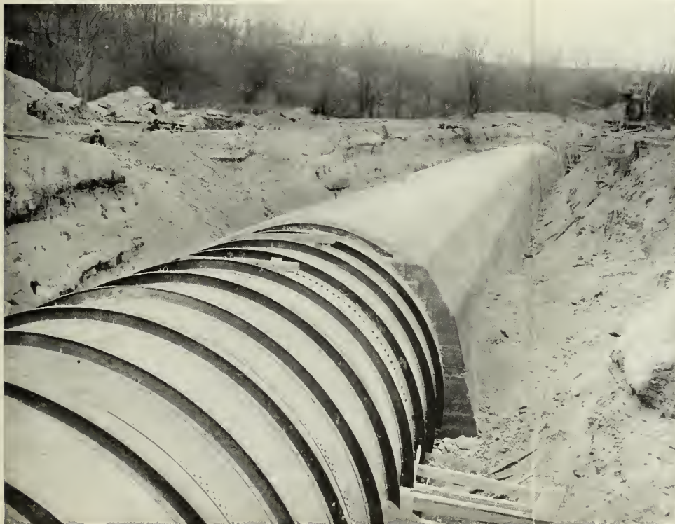
NO. 1 MAIN CONDUIT DURING CONSTRUCTION
