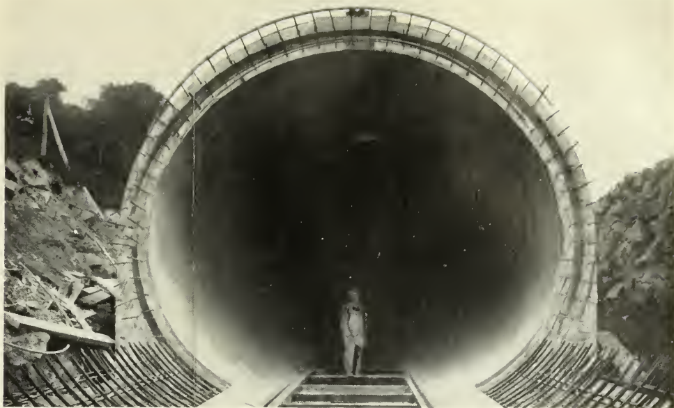
NO. 2 MAIN CONDUIT DURING CONSTRUCTION
