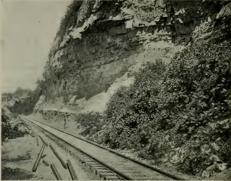
FIG. 5.—Showing extent of erosion at base of the Niagara shale since 1854. (See description in the text.)
