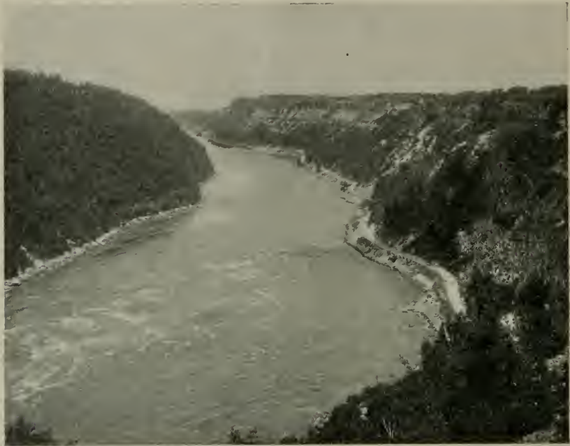
FIG. 1.—Looking north from below the Whirlpool, showing the electric road at the bottom of the east side of the gorge, and the steam road descending the face about halfway to the top.
