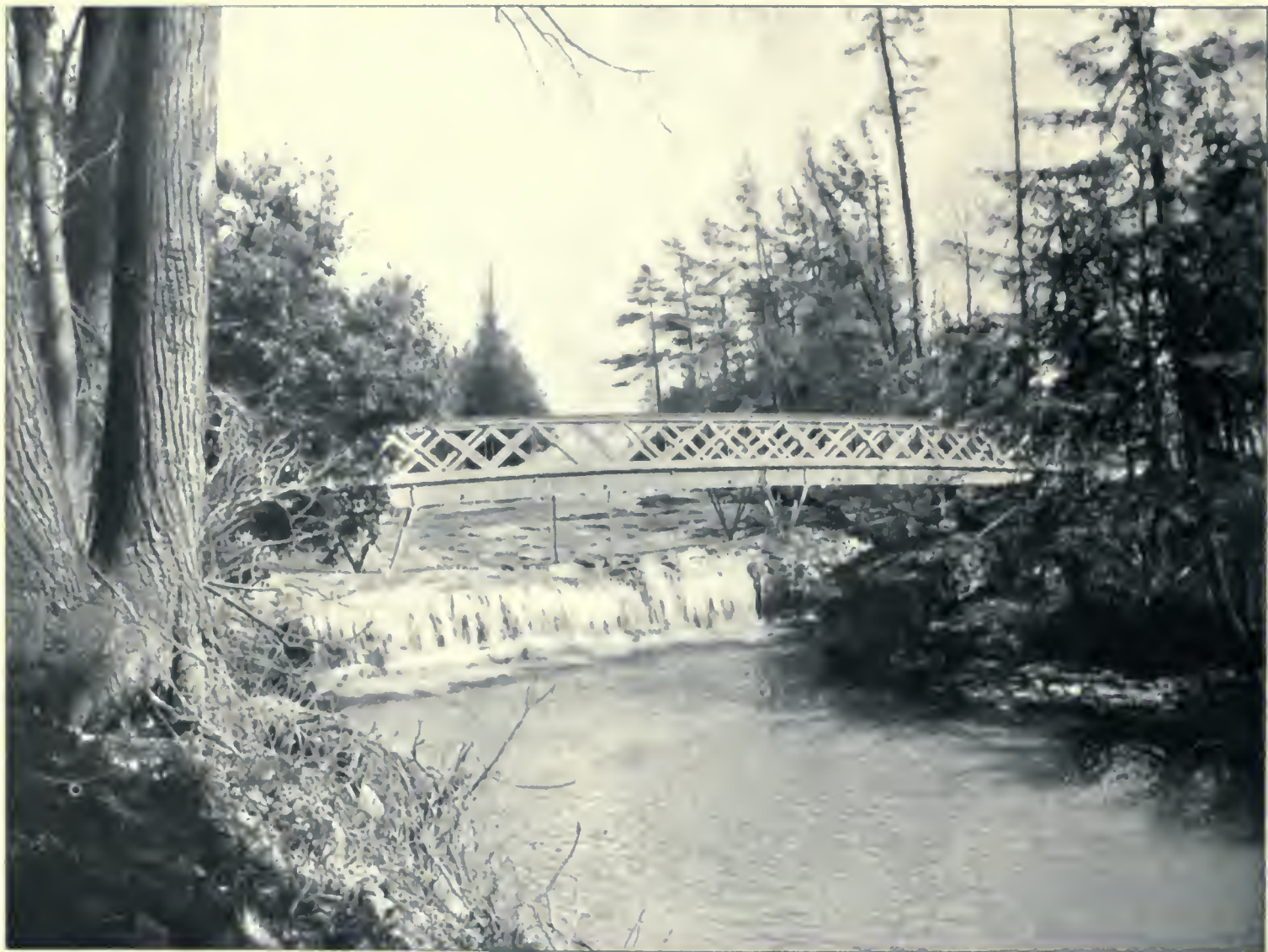
BRIDGE TO FIRST SISTER ISLAND.
