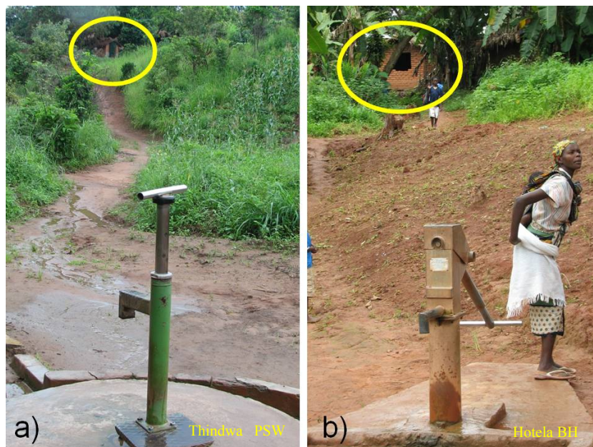
Figure 4 Protected shallow well (a) and borehole (b) located downhill from latrines/toilets
