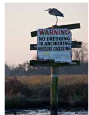
A sign warns of a pipeline crossing in Louisiana. Because of coastal erosion, many pipelines are closer to the surface and in some cases are even in open water. Photo: Paul Goyette
