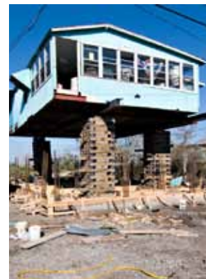
A house near Cocodrie, LA, is elevated as a defense against storm surge flooding. Photo: Paul Goyette
