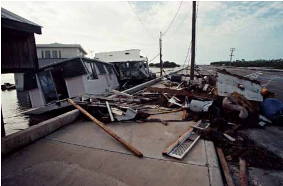
Houseboat Row on South Roosevelt Boulevard in Key West, FL, after Hurricane Georges in September 1998. Photo: Monroe County Public Library/The Dale McDonald Collection
