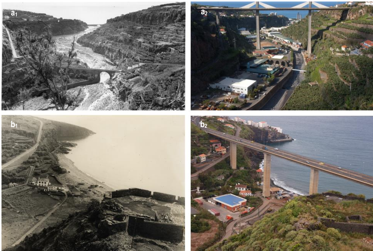
Figure 4.45 Construction over river bed and banks, and also over shore cliffs, especially in south coast. Ribeira dos Socorridos (a 1 ) in 1930s (Figueiras Photographers, AP), and (a 2 ) in 2010 (MS, AP); Porto Novo Cove (b 1 ) in first quarter of 20th century (unidentified photographer, ARM), and (b 2 ) in 2006 (AP, ZF).
