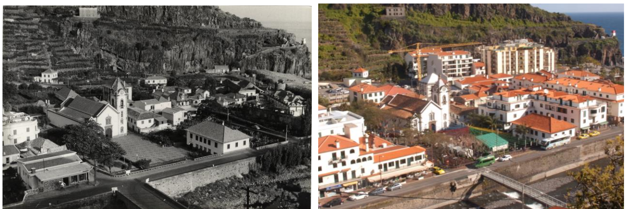
Figure 4.21 Historical and repeated photographs located in southern coast (Ribeira Brava) as an example of a pair exhibiting global landscape change under 50% (GLC = 21%), in which construction, agriculture and cliff faces showed high agreement between past and present landscape, being ultimately responsible for the low change level. Old photograph from early 1960s (by unknown photographer, ARM) and new one taken in 2011 (AP, MB).
