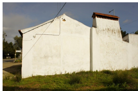
Fig.4. Monitored facade (West facade).
