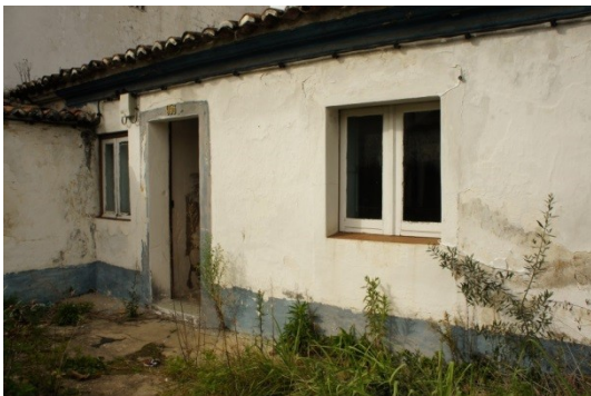
Fig.6. Monitored façade (South façade). probes' location.
