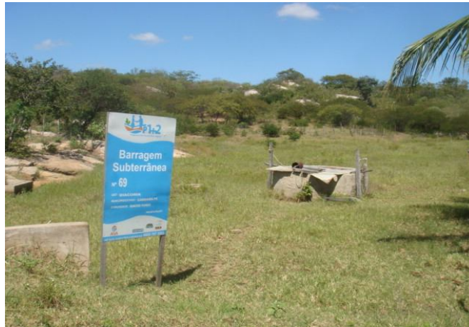
Figure 6 - Underground dam, Afogados da Ingazeira municipality, Pernambuco state, Brazil.
