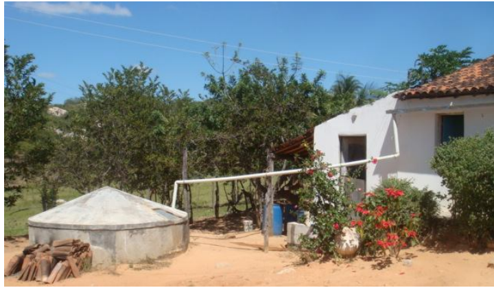
Figure 2 – Conventional cisterns. The rainwater is collected on a house roof and led through a gutter into a cistern. Afogados da Ingazeira municipality, Pernambuco state, Brazil.
