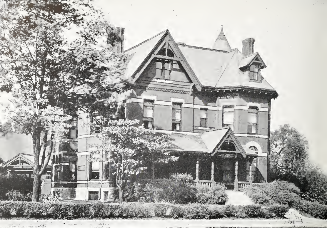
Administration—1204 North Delaware Street
