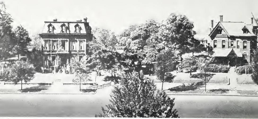
View of the Delaware Street Campus.
