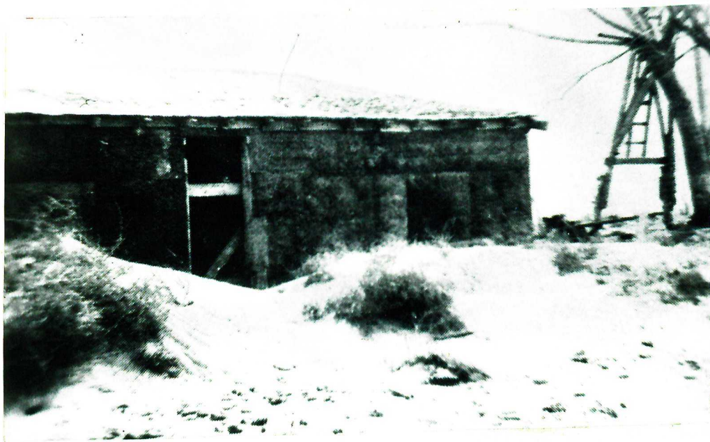
FIGURE 5. A typical result of destructive wind erosion.
