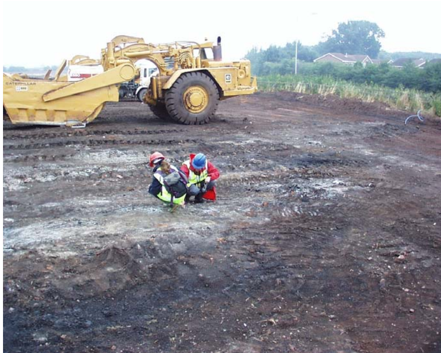
b. Soil mixed with coal measures mudstone, brick and coal at shaft.
