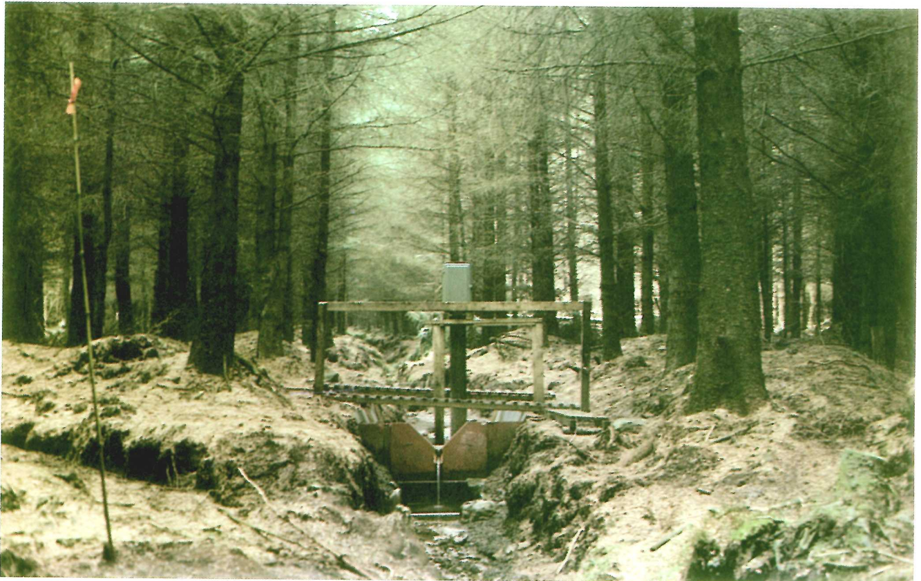
Plate 2. A weir on a drainage ditch at Kershope Forest. Joint research work by the Forestry Commission and the Institute of Terrestrial Ecology is leading to an understanding of the effects of coniferous forests on drainage water. (Photograph J K Adamson)
