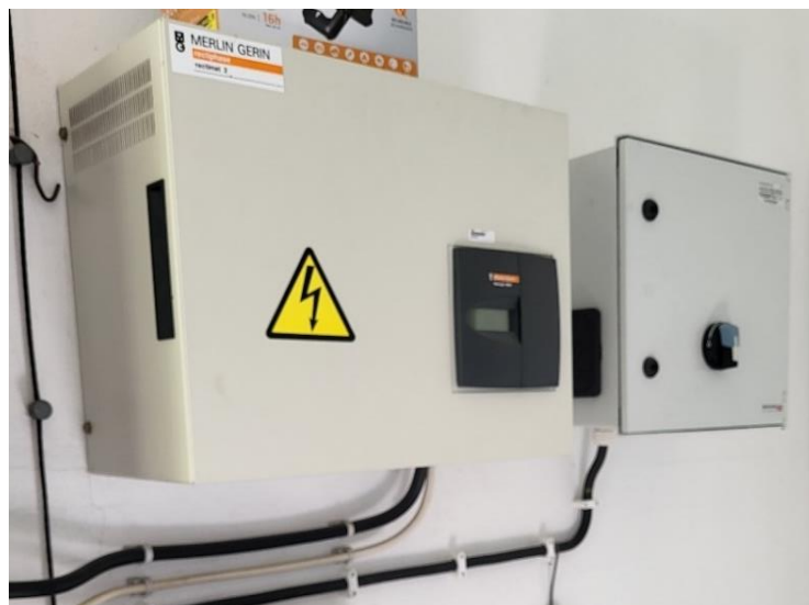
Figure 4.14 – Condenser bank PT2.
