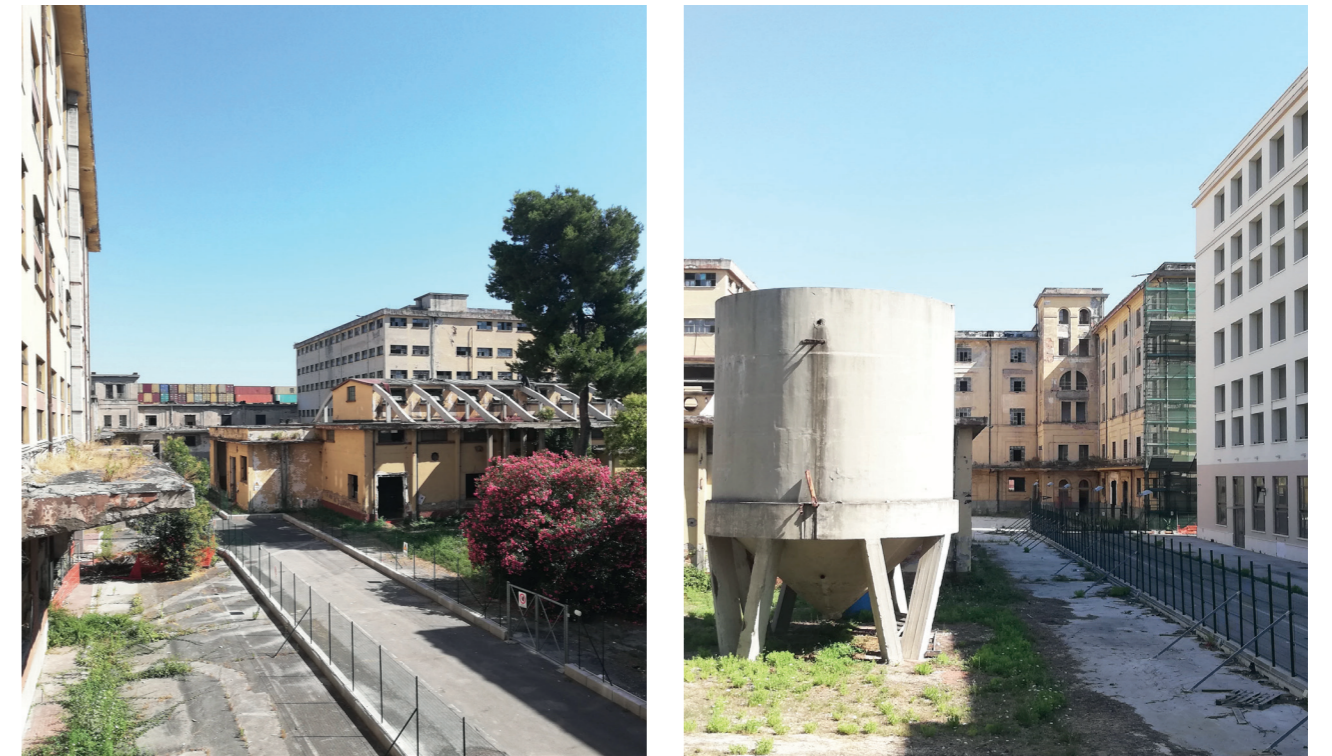
Figure 4: Current condition of the ex Manifattura Tabacchi. Source: photo by the authors.
