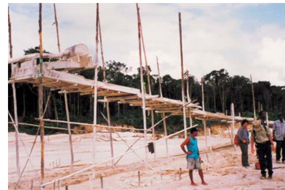
Plate 1 Large sluice (Guyana).
