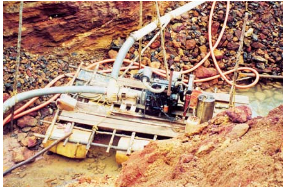
Plate 5 Large 6 inch gravel pump (yellow) powered by a diesel engine (Guyana).
