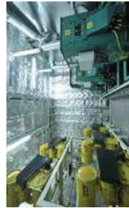
Sound protected machine room with Feed Blowers and generators.
