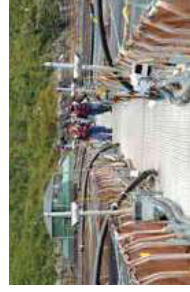
The wide walkways provide superior support for predator nets, well spaced from the fish net. This is a crucial feature for some areas.
