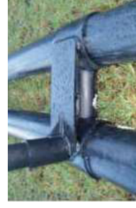
Forget corrosion! Polarcirkel bracket after 10 years in saltwater!
