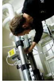
The Air Control unit is installed between the Air-Cooler and Feed Doser Valve.
