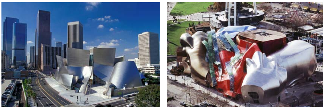
Ilustración 23. Frank GEHRY, [Izquierda] Walt Disney Concert Hall , Los Angeles, 2003. [Derecha] Experience Music Project (EMP) , Seattle, 2000.
