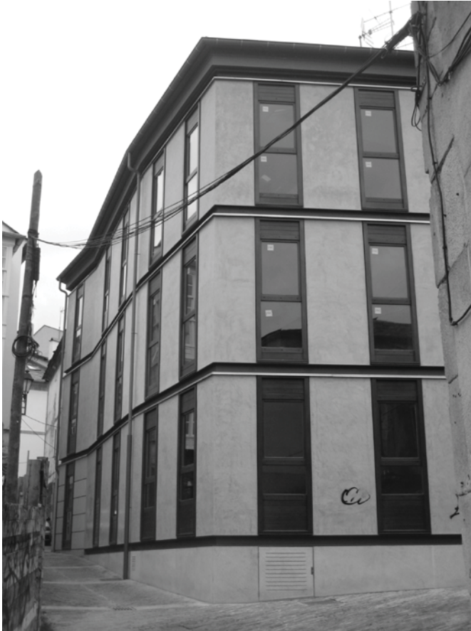
Figure 5. Housing in Rúa Falcón upon completion.
