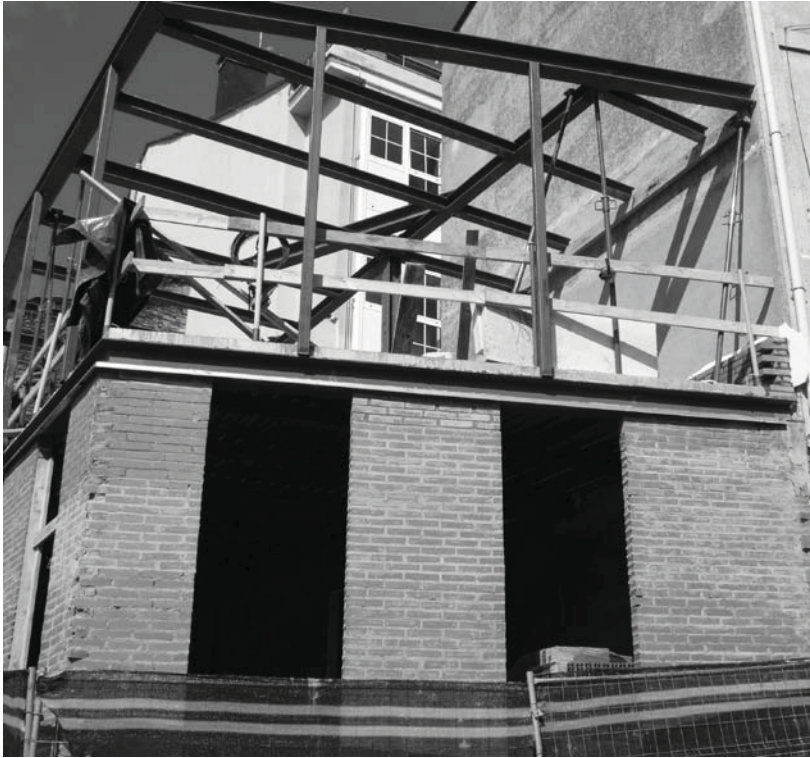
Figure 6. Housing in Rúa Falcón under construction.
