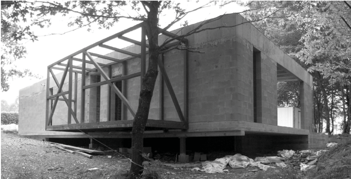
Figure 2. The building under construction.
