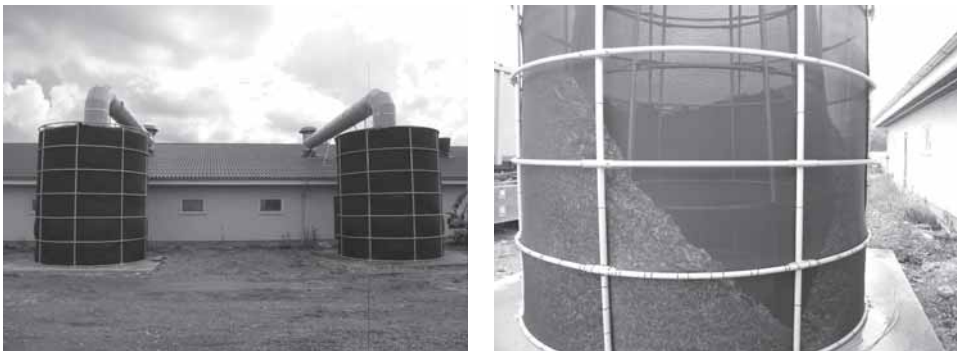
Figure 1. Design of the vertical biofilters.
