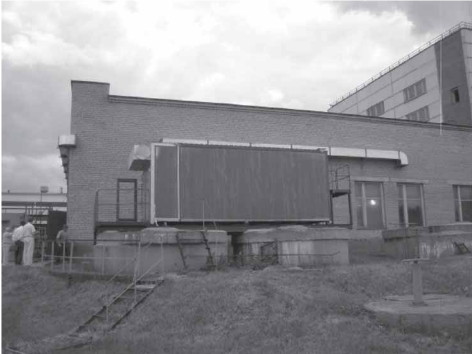
Figure 2. Biofilter at the premises of Moscow Water Works.
