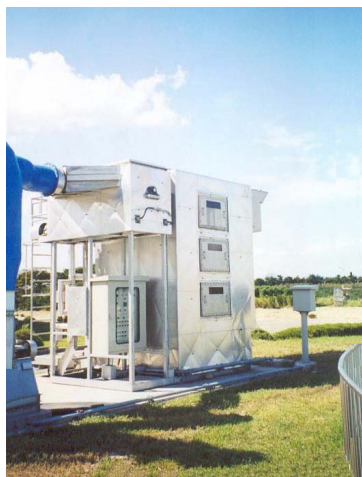
Figure 3. Trickleing bioreactor for air deodouration. Module with a capacity of 12,000 m^3/h and recommended EBRT of 3-3.5 s.
