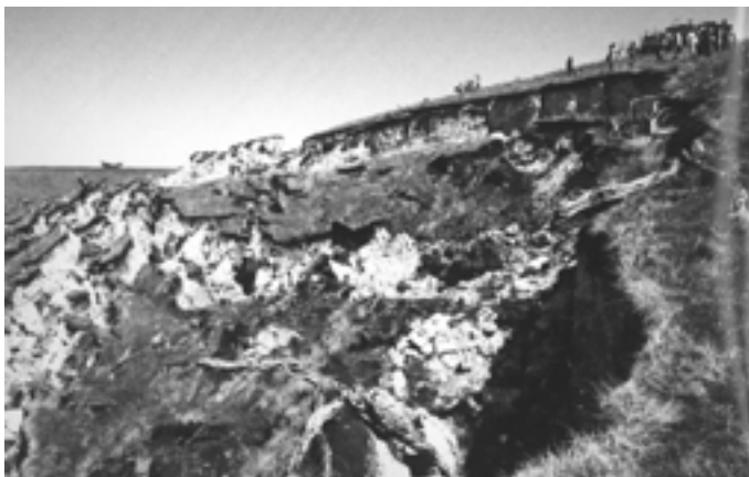
Figure 9b. Tension crack at head of Landslip, 1974.
