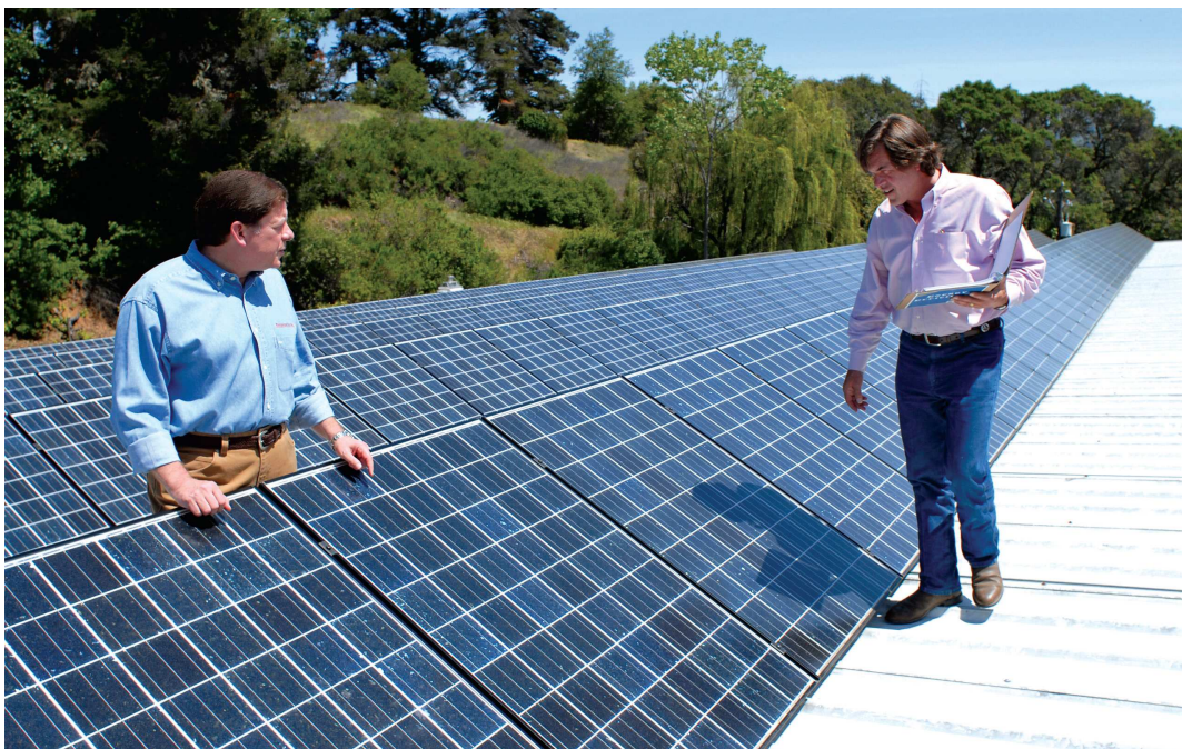
Figura 5 Paneles fotovoltaicos en Parducci Wine Cellars, California 10
