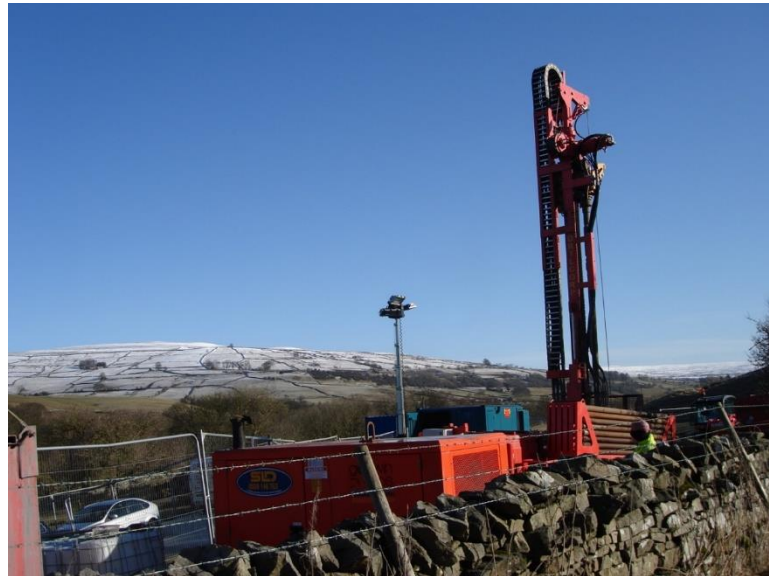
Figure 9 Eastgate 2 drilling operations, 1st March 2010 (photo by Jon Gluyas).
