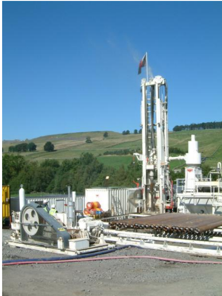
Figure 6 Eastgate drill rig (photo by Paul Younger).
