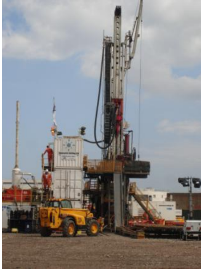
Figure 13 Science Central drilling rig July 2011 (photo by Jon Gluyas).
