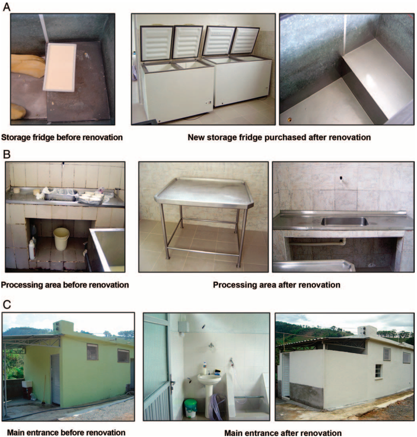
FIG. 2. Photographs of plant F before and after renovations. (A) Coolers used for storage of MFC. (B) Cheese processing area. (C) Main entrance.
