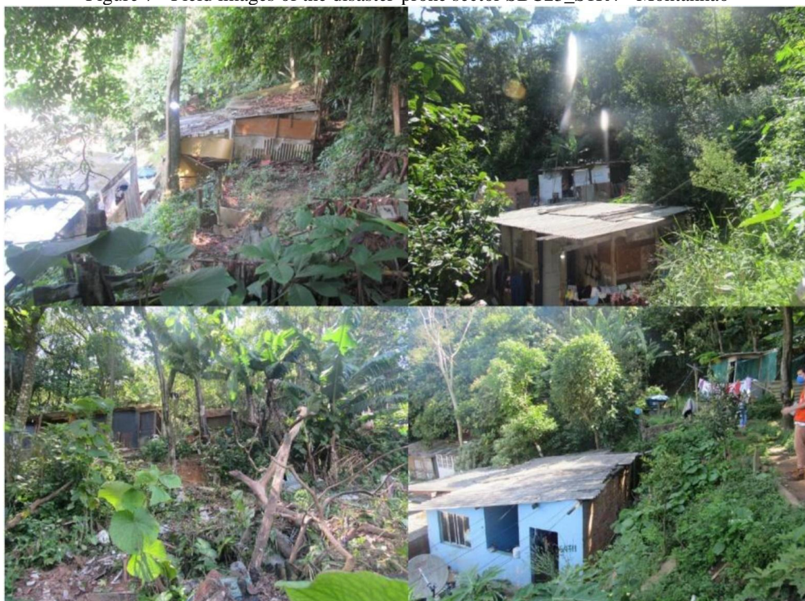
Figure 7 - Field images of the disaster-prone sector SBC23_S1R4 - Montanhão
