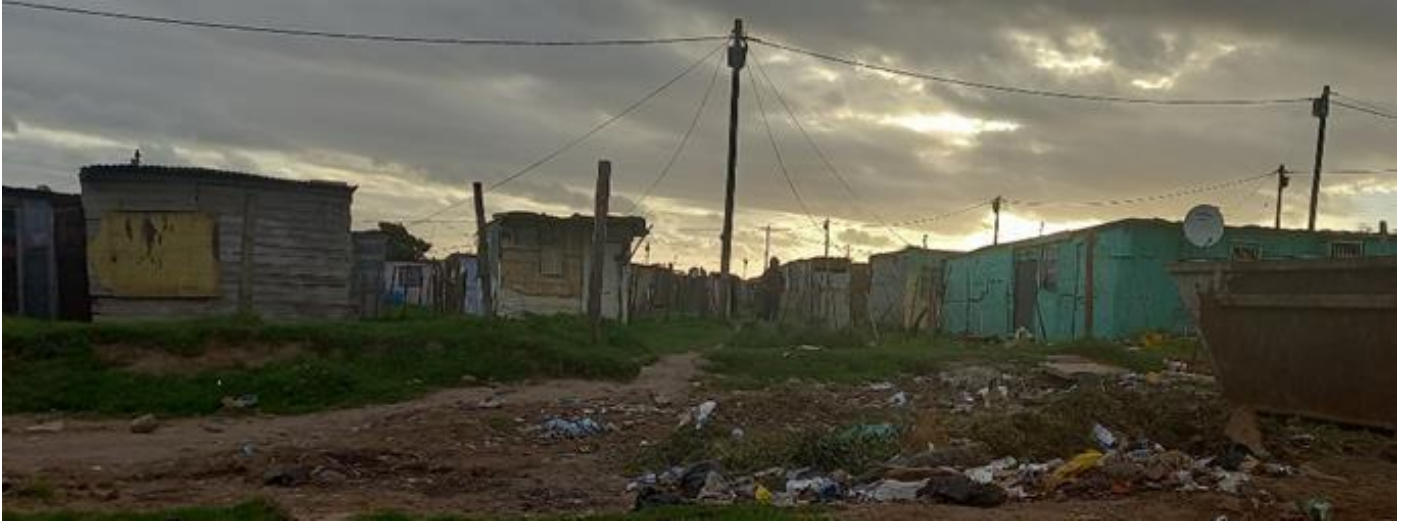
Fig 1.2.: A picture of the toilets used in one of the residential areas in the study area next to one of the dumping sites where CWP general workers work (Source: the picture was taken by the researcher during a site visit conducted in November 2021)
