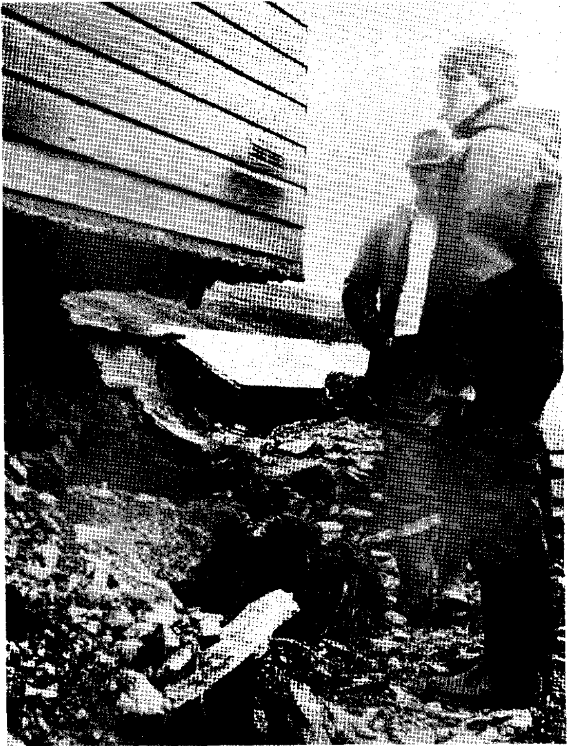
Plate 20. Undermining of Gwy flume hut by overtopping flood waters.
