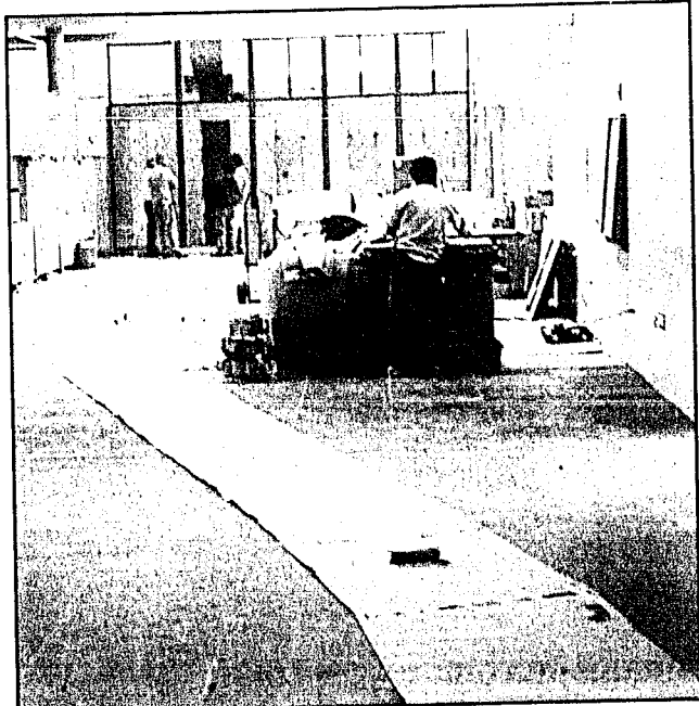
The new racquetball courts are almost ready to see some action (above). Construction personnel work on some of the last details in the front desk area (left). Bricks hold down the edges of the new sports floor while the glue dries (far left).
