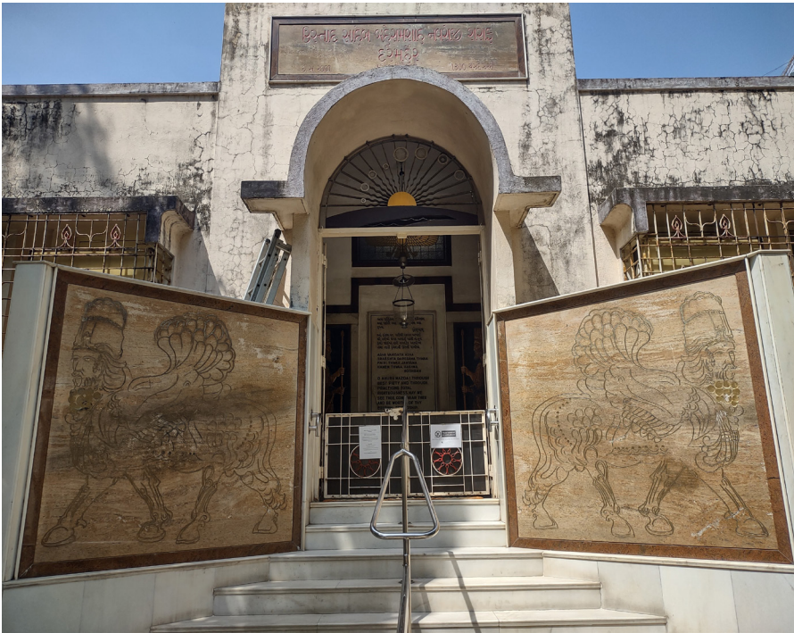
Fig. 2. Ustad Saheb Behramshah Nowroji Shroff Daremeher fire temple, Mumbai, India, 2023. Photograph © Mariano Errichiello.
