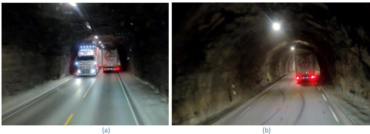
Figure 7. (a). Tight passage when encountering oncoming truck. (b). Narrow tunnel without centerline. Both seen from truck 3.
