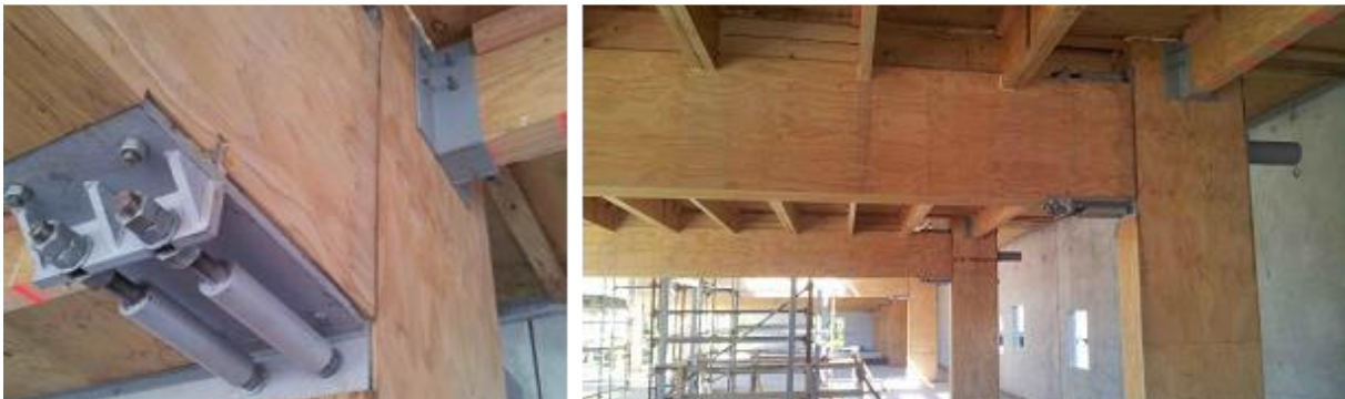
Figure 11: Merritt Building beam-column connections
