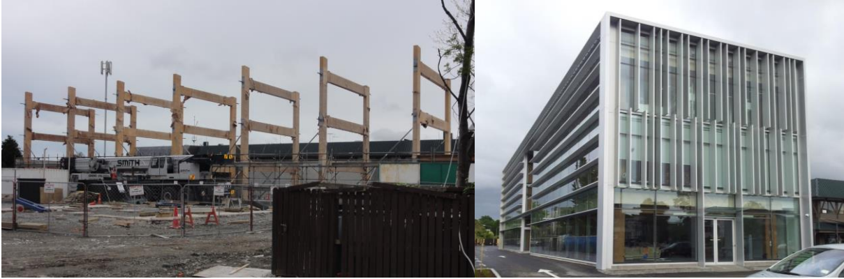
Figure 10: Merritt Building frames and completed building
