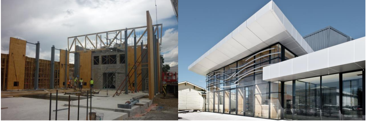
Figure 7: Carterton Events Centre during construction and after opening
