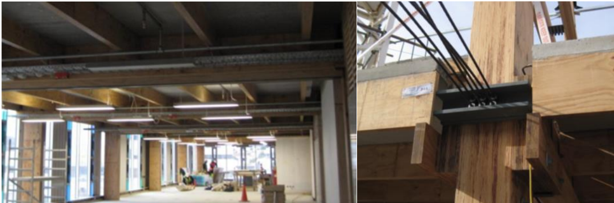
Figure 9: CoCA Building floor and post-tensioning anchorage
