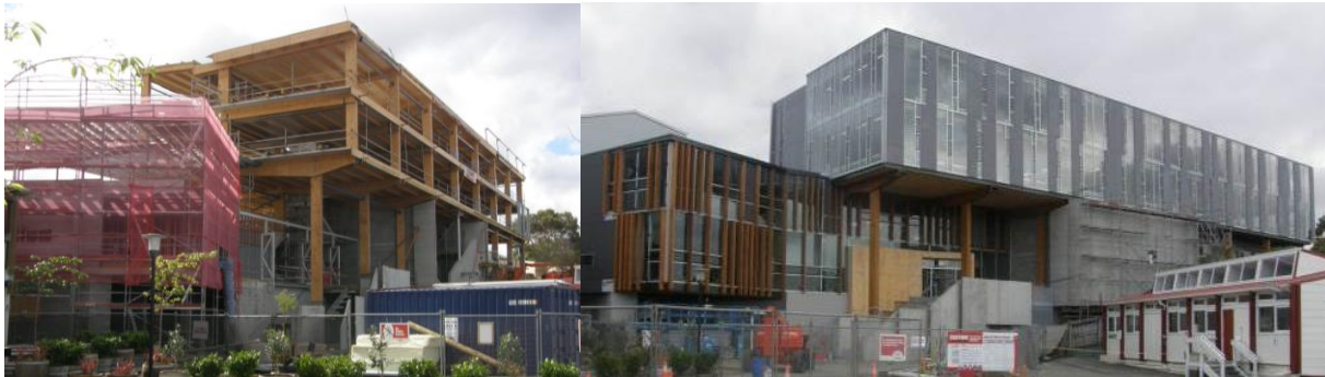
Figure 8: College of Creative Arts during construction and completed
