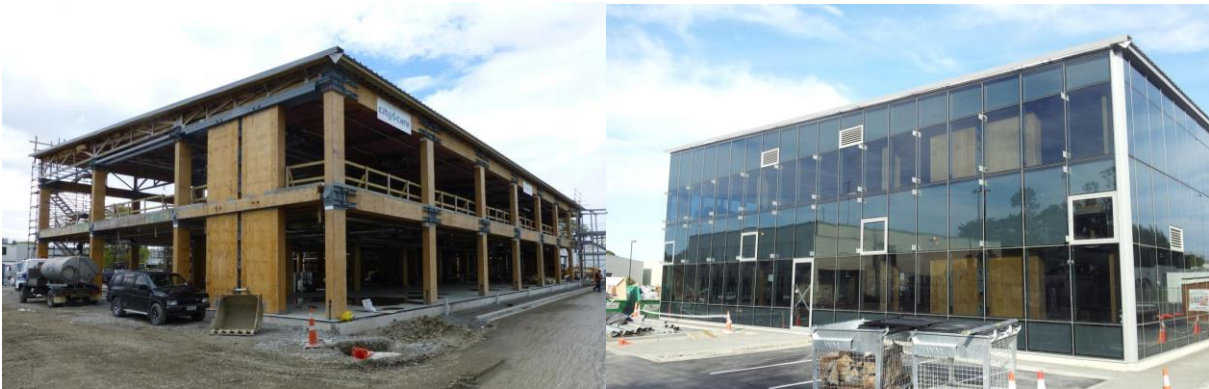
Figure 12: Trimble Building structure and completed building
