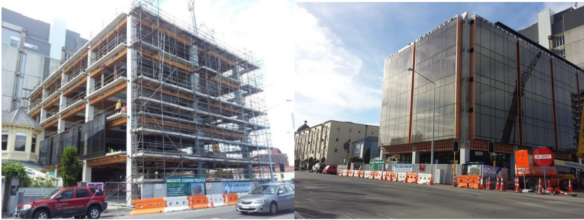
Figure 16: St Elmo Court structure and completed building
