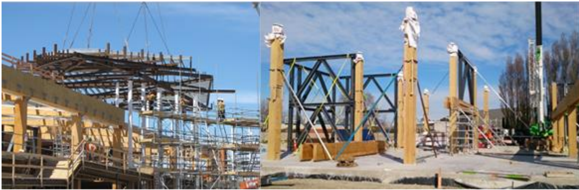
Figure 17: Tait Communications complex structure during construction
