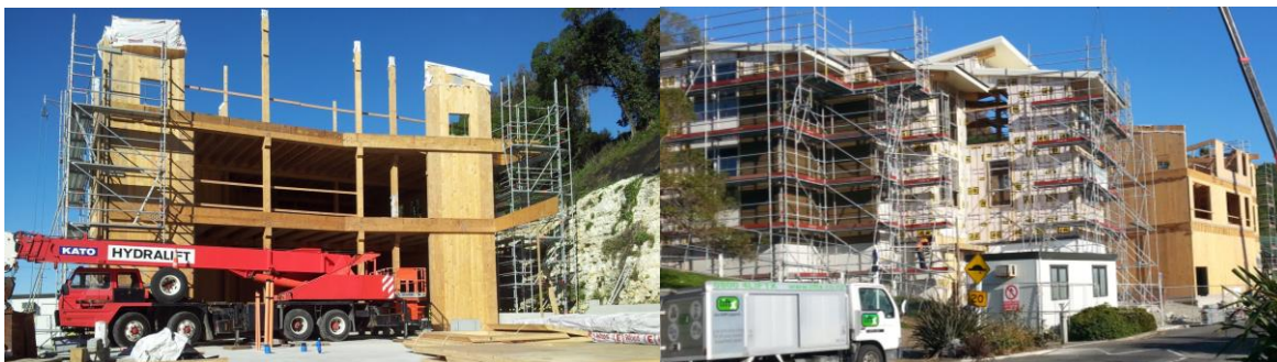
Figure 15: CLT Shear walls within wooden structure of Kaikoura District Council Building
