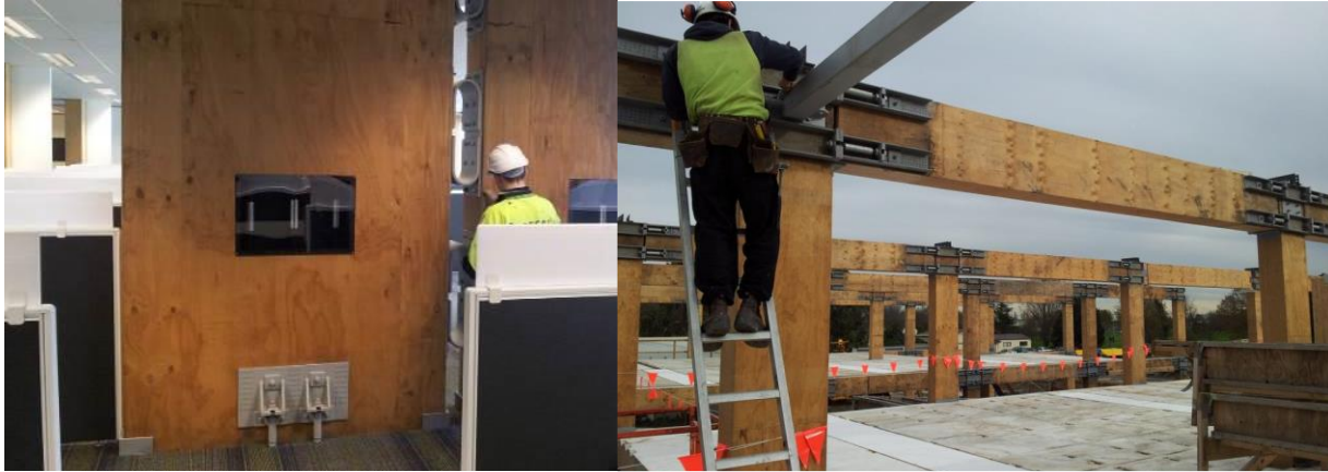
Figure 13: Walls and Beam-Columns with energy dissipating connections in Trimble Building
