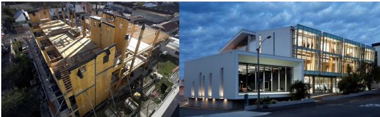
Figure 5: NMIT Arts and Media Centre during construction and after completion
