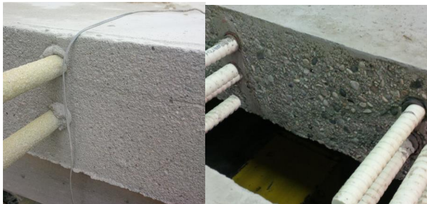
Figure 11: Previous sandblasted surface (left) and the new coarse aggregate finish (right).
