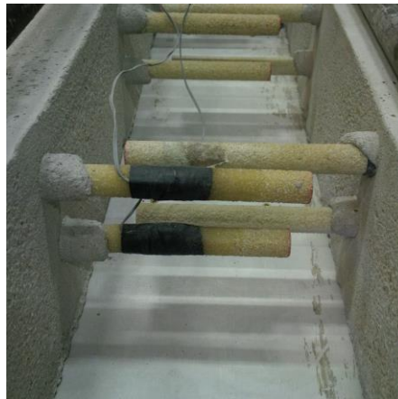
Figure 3: Closure strip prior to UHPC placement.
