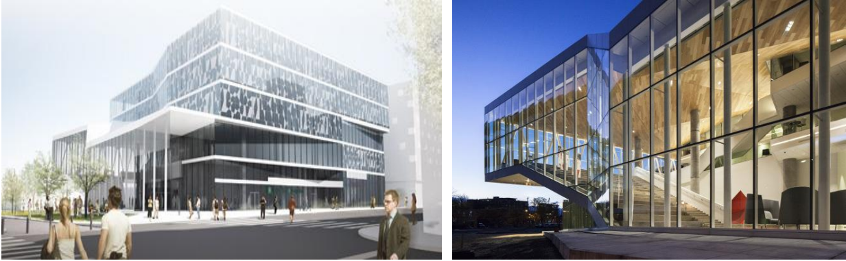
Figure 1: General 3-D views of the MDE Building in the finished phase a) North view reproduced from drawings, b) South-East facade with steel cantilever (Reproduced from Carignan (2015))
