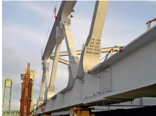
Figure 1: Metallized Memorial bridge, Kittery, ME & Portsmouth, NH (Credit: Canam-bridges)
