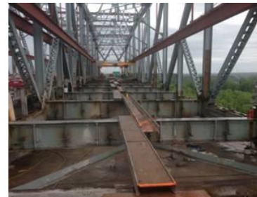
Figure 4: Structural Steel prior to Deck Panel Installation
