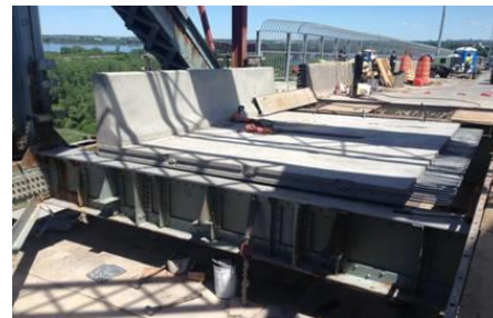
Figure 6: Precast Concrete Panel Installation
