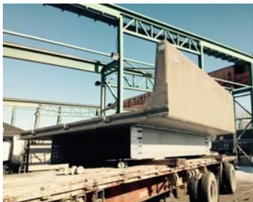
Figure 5: Deck Panel Transportation
