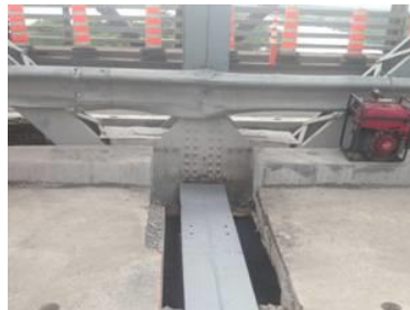
Figure 3: Strengthening of Existing Floor Beam
