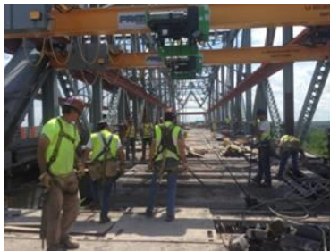
Figure 2: Existing Deck Demolition
