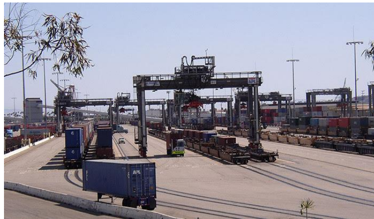
Figure 13: Rail-mounted train stacking cranes (Source: Tirschwell 2015)
