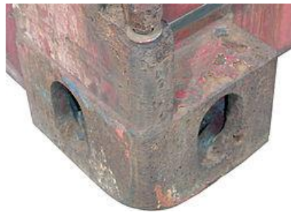
Figure 8: Corner fitting
