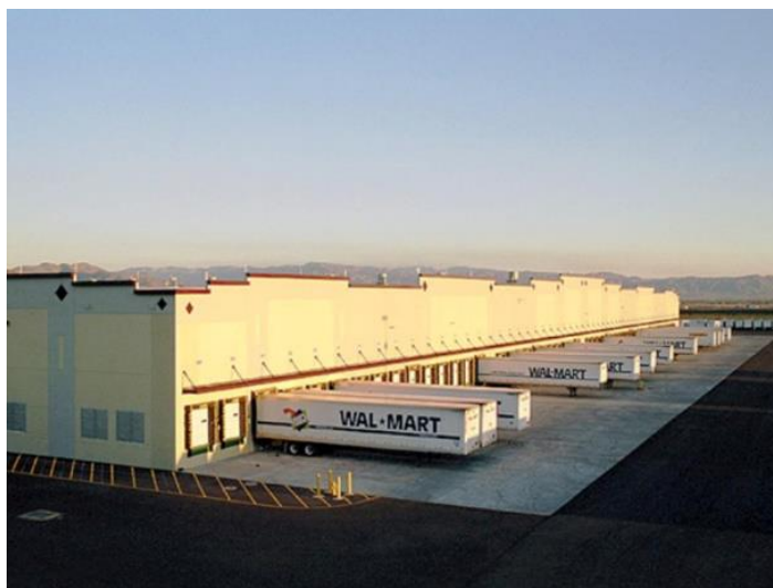
Figure 25: Walmart distribution center truck docks (©Blue Scope Construction)
