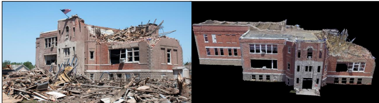
Fig. 3: Damaged Wisner-Pilger Middle School: ground-survey image (left) and point-cloud imagery (right).
