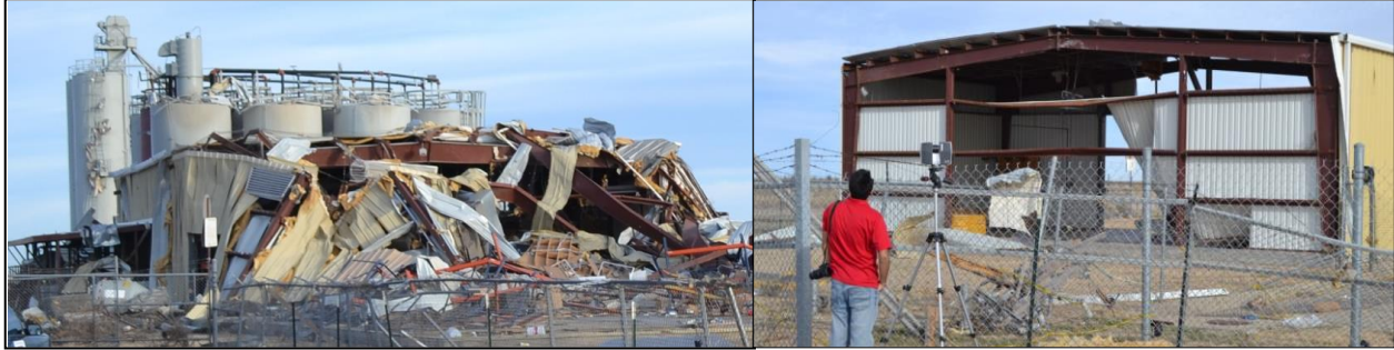
Fig. 4: Tornado damage to Halliburton facility, Pampa, TX.
