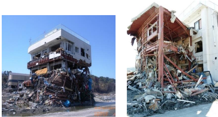
Figure 1: Debris impact on structures following the 2011 Tohoku Japan Tsunami (Nistor, 2011).
