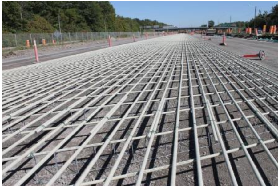
(b) Transverse and longitudinal bars
