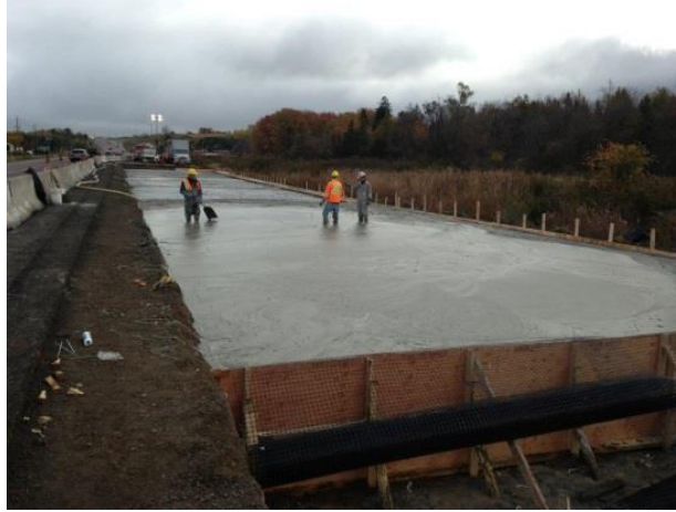
Figure 4: Geogrid Installation
