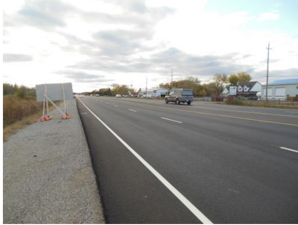
Figure 5: Completed pavement, one year after construction
