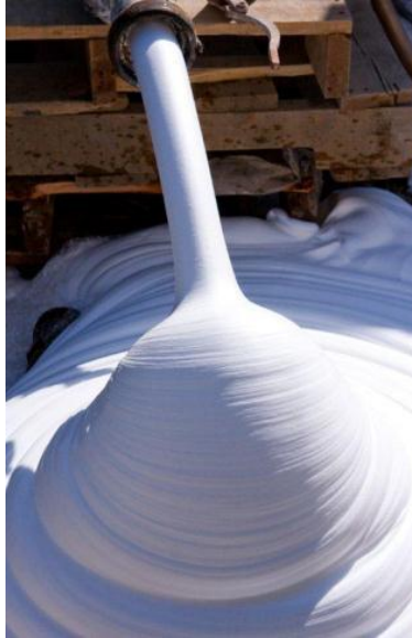
Figure 1: Foamed cellular concrete being discharged from a pipe
